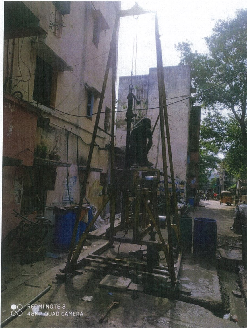
Figure 2 b): Images were taken during the site investigation
