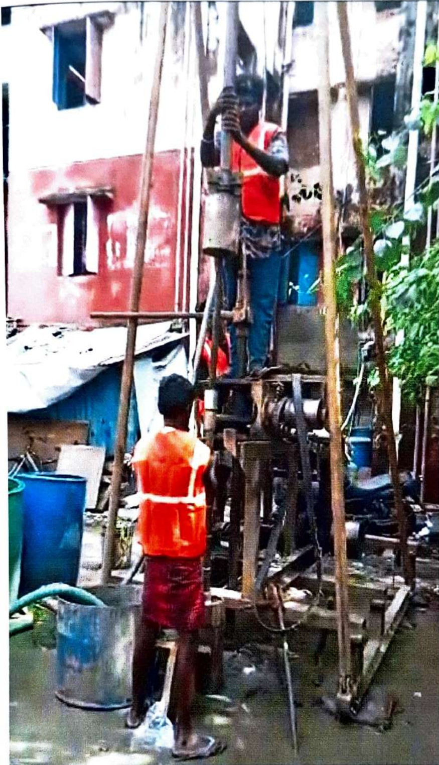
Plate 1 SPT test is in progress at Reconstruction of Tenements (S+13 Floors) in Ward No. 52, Zone V, Chetty Thottam, Chennai - 600 013.
