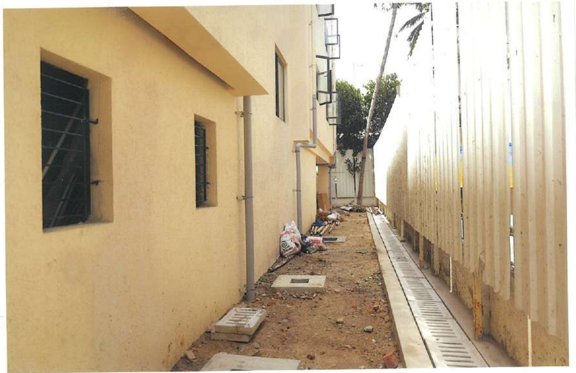
STILT FLOOR (SOUTH SIDE)
