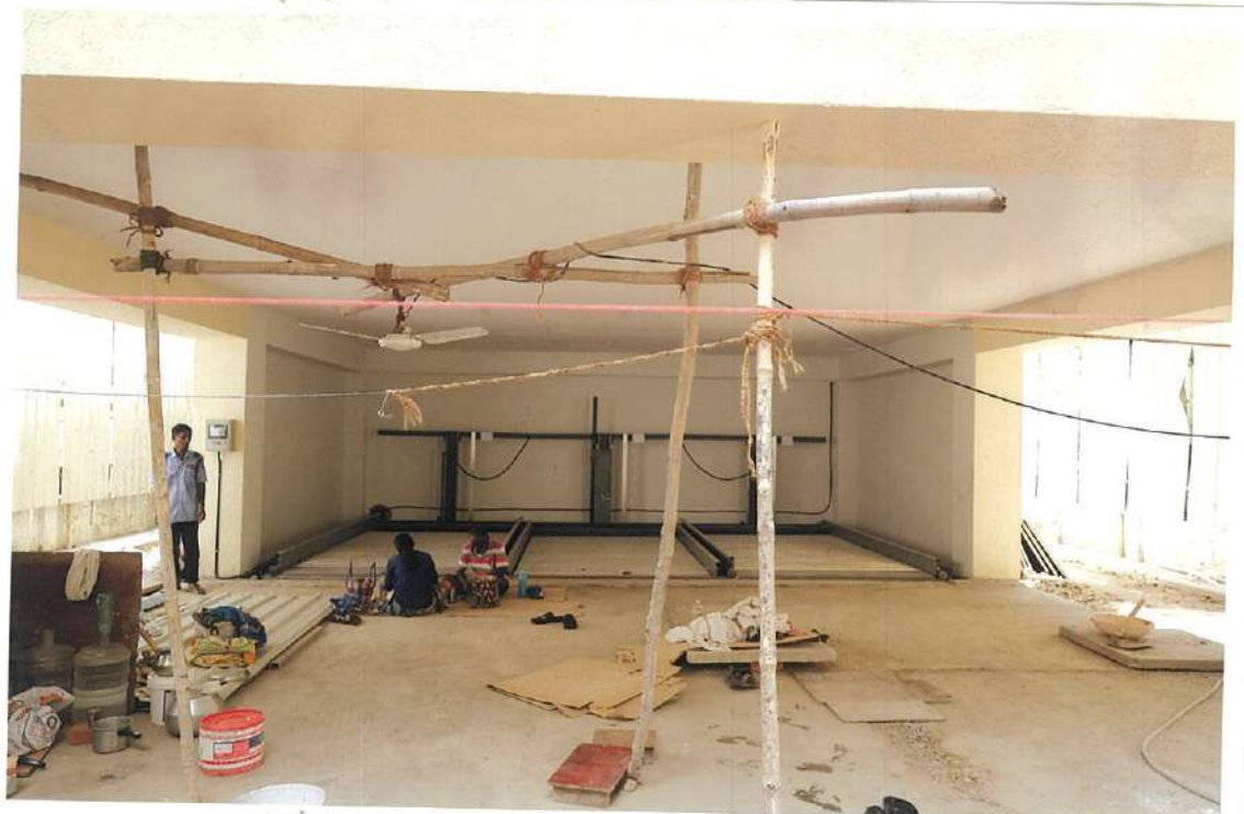
REAR SIDE PARKING AREA (EAST SIDE)
