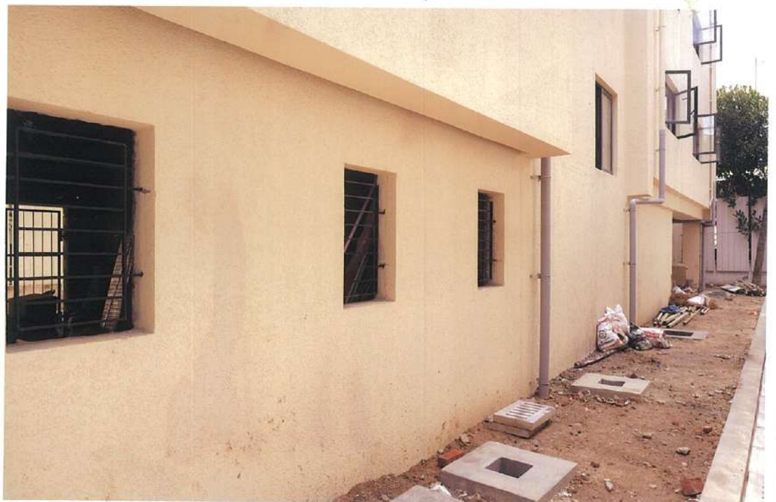
STILT FLOOR (SOUTH SIDE AREA)
