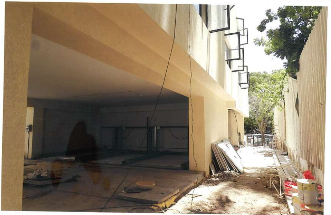
NORTH SIDE STILT FLOOR PARKING AREA
