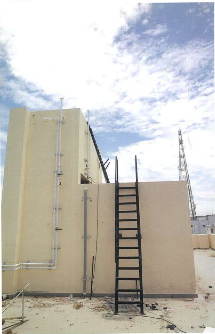
OHT AREA (TERRACE FLOOR)
