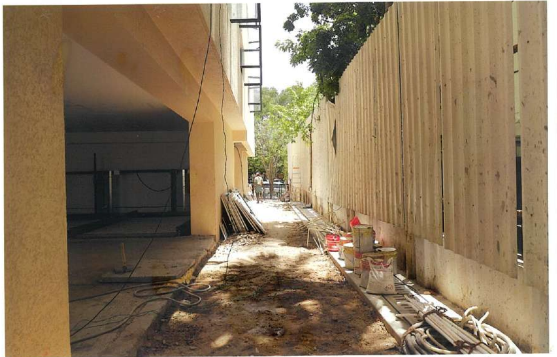
NORTH SIDE STILT FLOOR PARKING AREA
