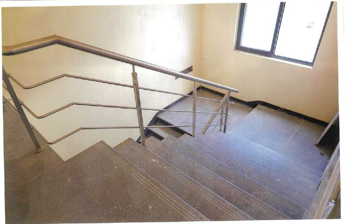
STAIRCASE RAILING (mid landing level)
