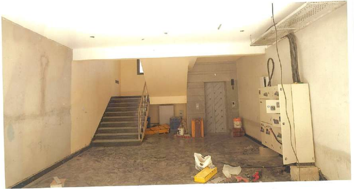
STILT FLOOR LIFT & STAIR LOBBY AREA
