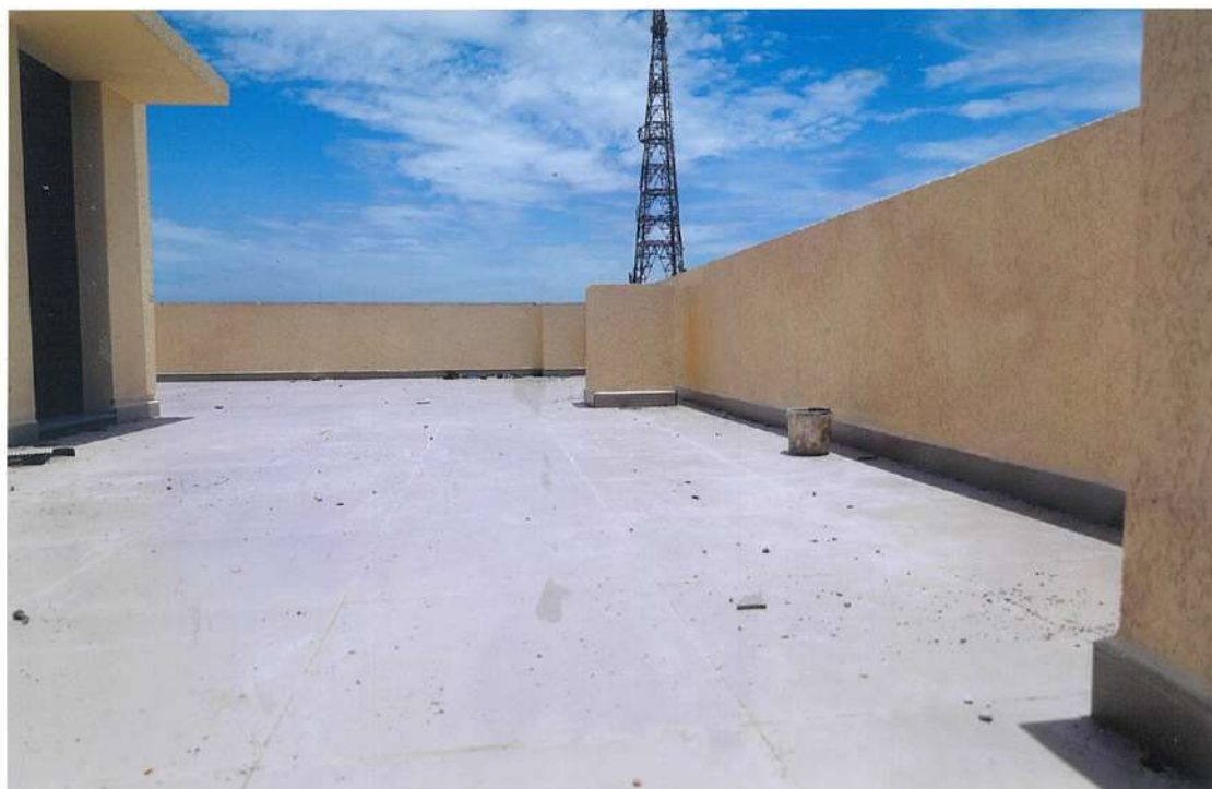
TERRACE FLOOR PARAPET WALL
