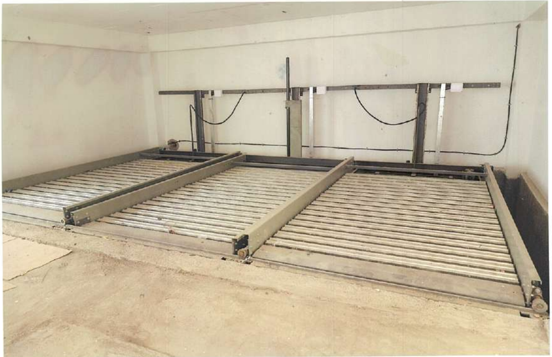
MECHANICAL PARKING IN STILT FLOOR
