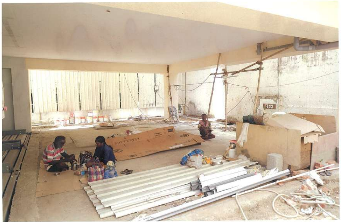
SOUTH SIDE STILT FLOOR PARKING AREA
