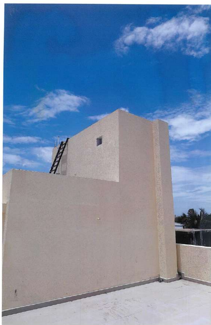
HEAD ROOM MACHINE ROOM WITH TANK
