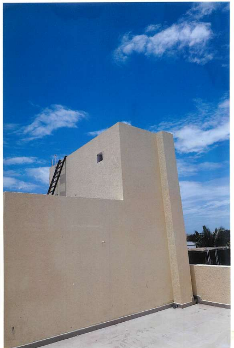
HEAD ROOM LMR TANK
