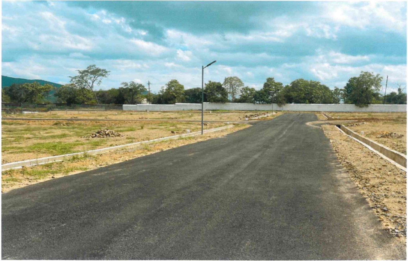
AFTER SHIFTING OF EB LINE
