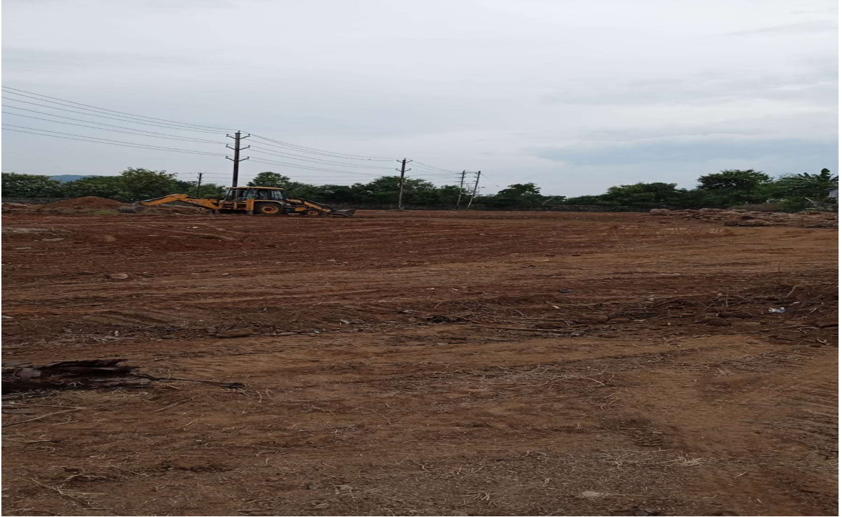
BEFORE SHIFTING OF EB LINE
