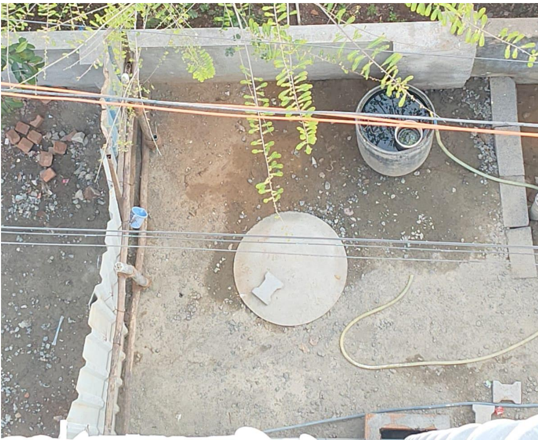
Rain water harvesting
