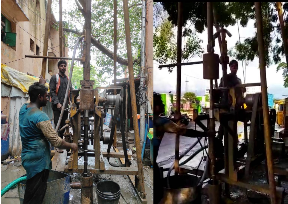
Plate 1 SPT test is in progress at the Reconstruction of Dilapidated Slum Tenements at Cox Colony Tenemental Scheme in Corporation Division 63, Zone V of Greater Chennai Corporation.
