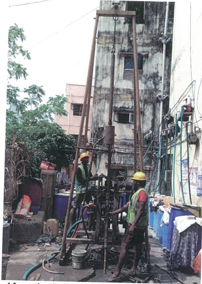
Figure 1 Geo-technical Investigation is in progress at Reconstruction of Tenements at North Giriappa Road Old in Zone IX, Division V, Greater Chennai Corporation.
