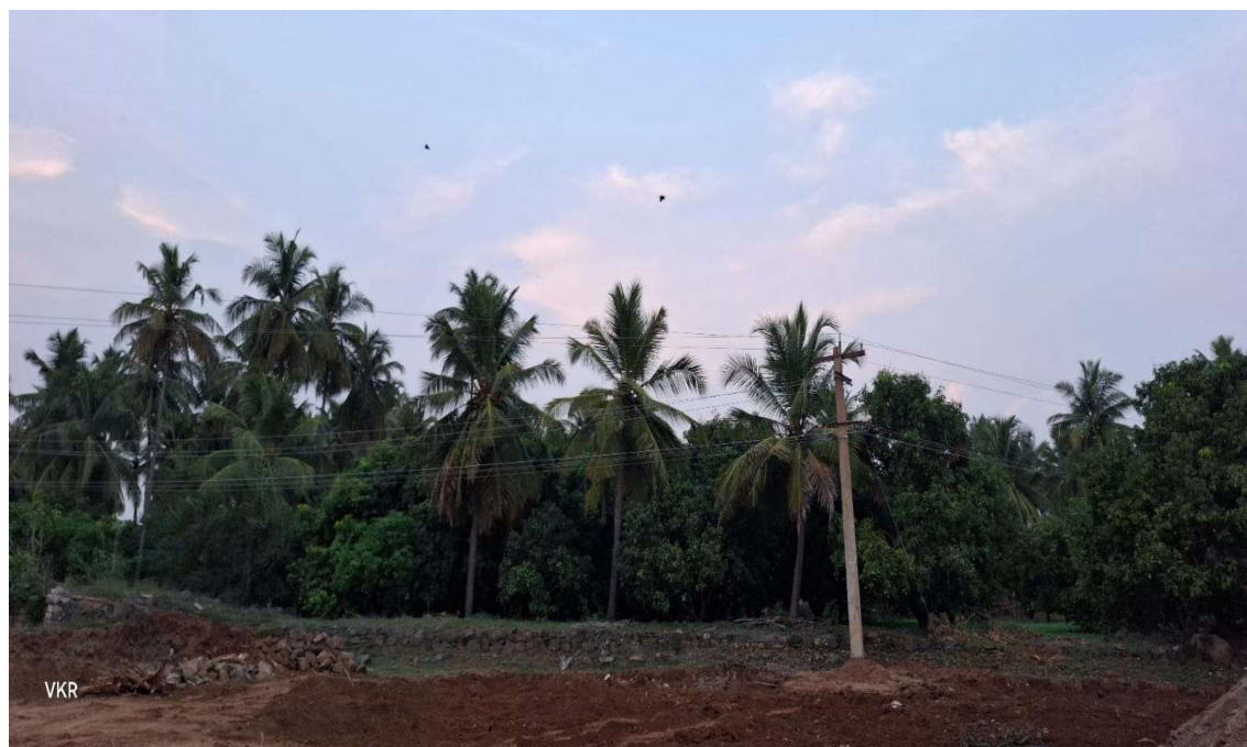
EB LINE BEFORE SHIFTING
