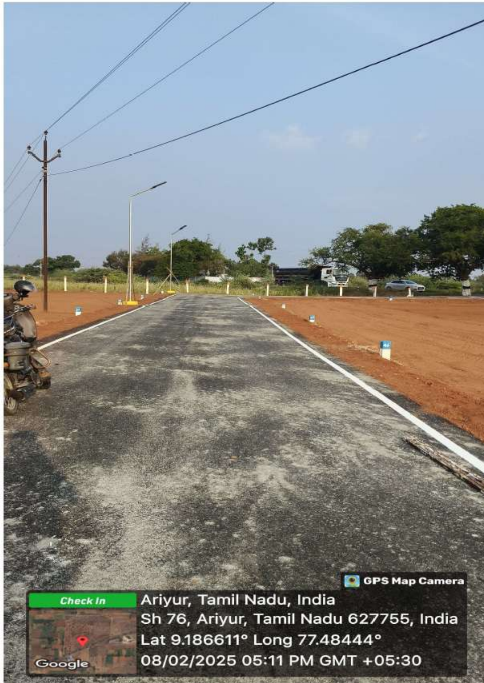
Photo before Removing EB Line`
