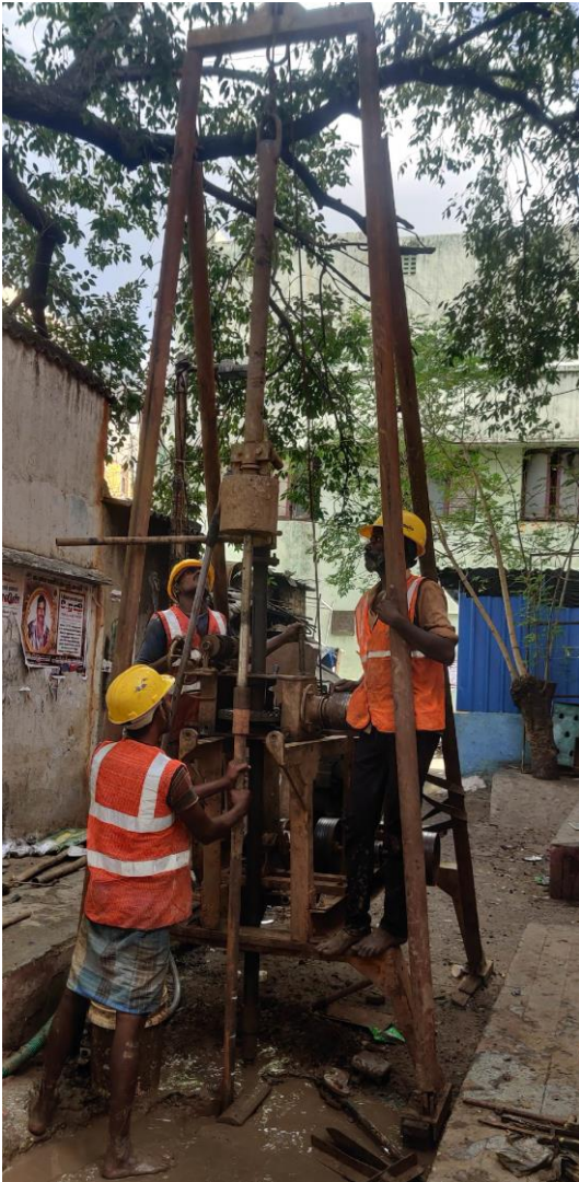
Plate 1 SPT test is in progress at the Proposed Reconstruction of Dilapidated Slum Tenements (S + 5 Floors) at Ellispuram Tenemental Scheme in Corporation Division 59, Zone V of Greater Chennai Corporation.
