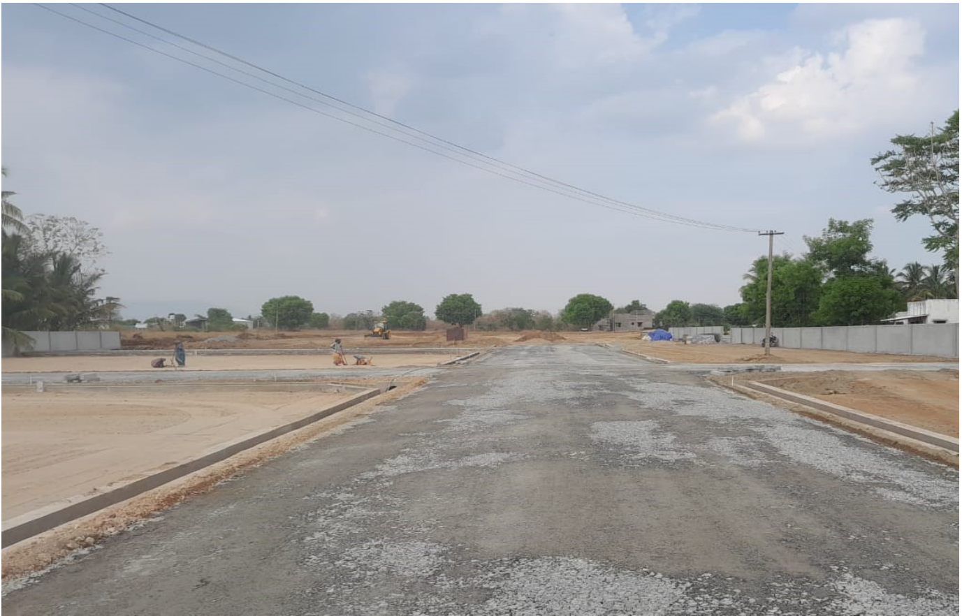
BEFORE SHIFTING OF EB LINE
