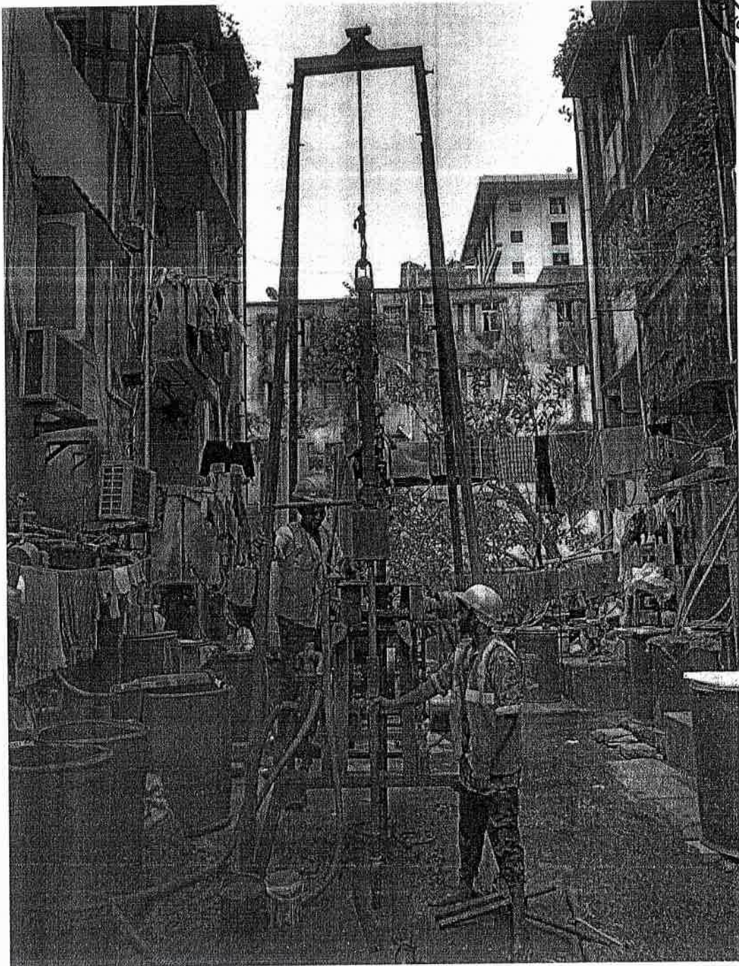
Figure 1 Geo-technical Investigation is in progress at Reconstruction of Tenements at North Giriappa Road Old in Zone IX, Division V, Greater Chennai Corporation.
