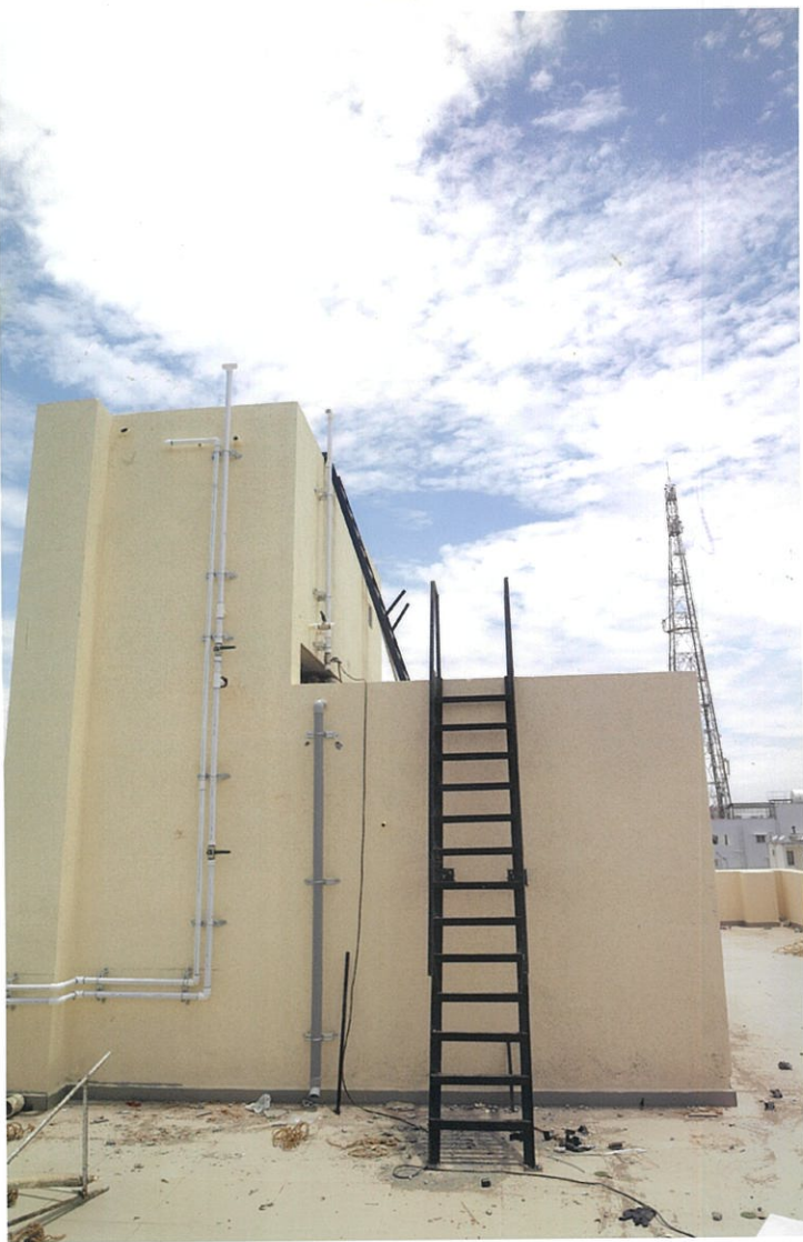
OHT AREA (TERRACE FLOOR)
