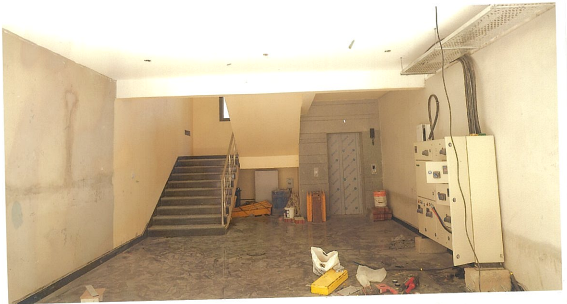
STILT FLOOR LIFT & STAIR LOBBY AREA
