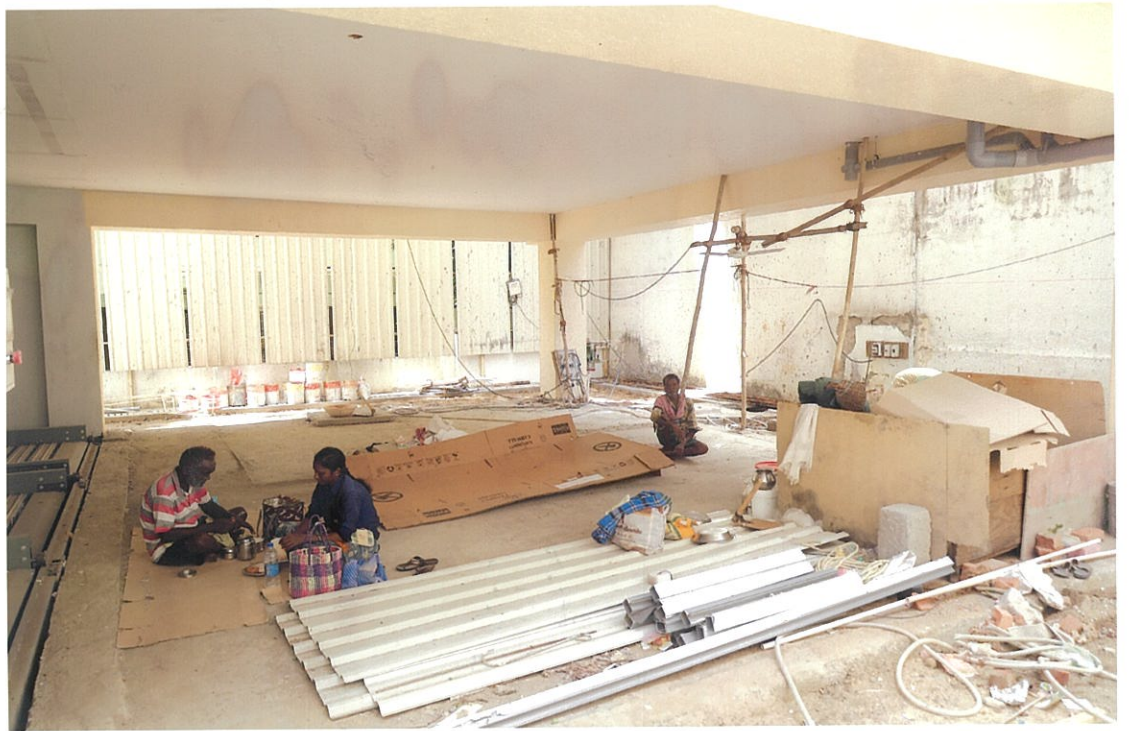
SOUTH SIDE STILT FLOOR PARKING AREA
