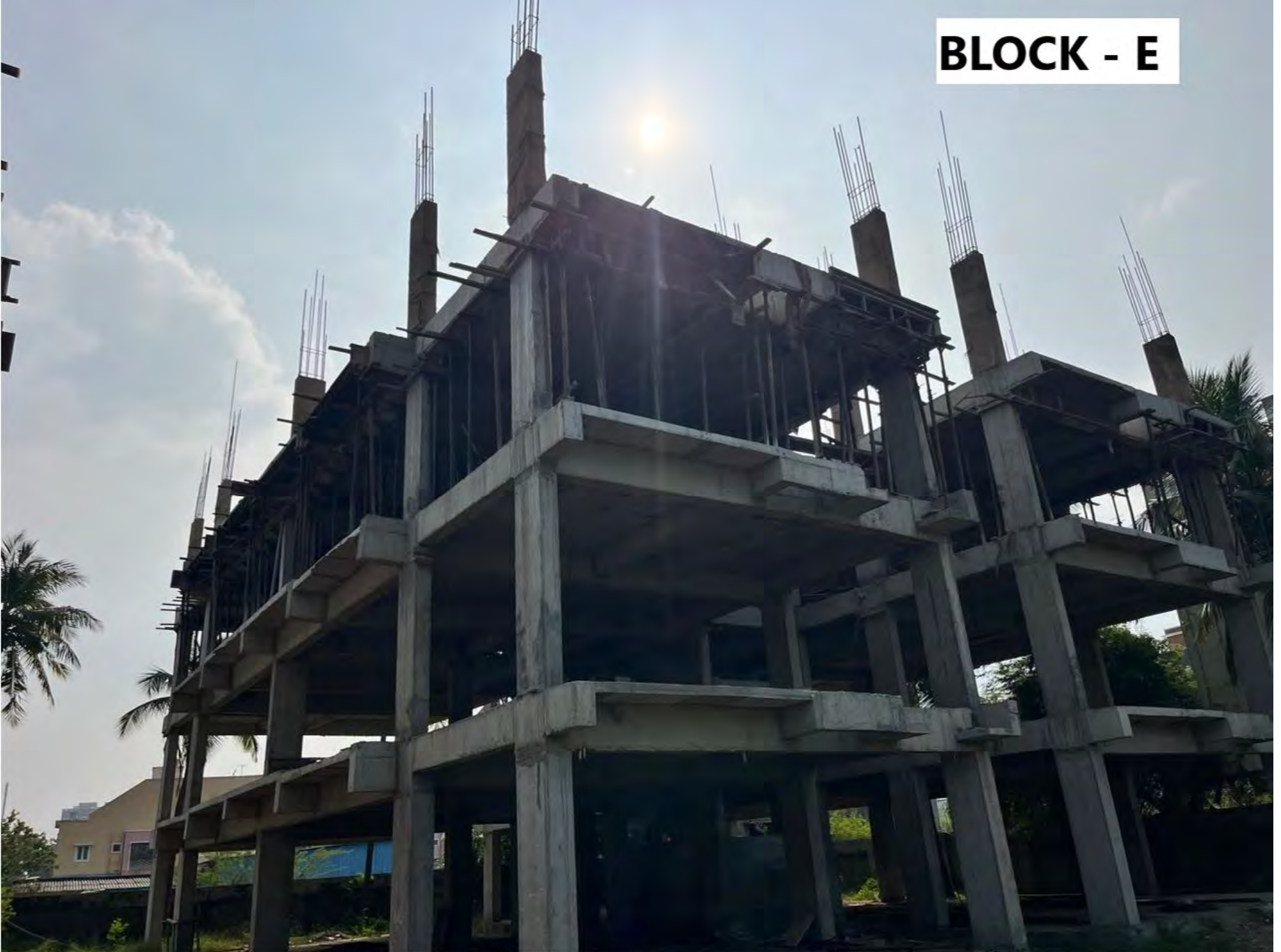
3rd Floor Column concrete completed, Shuttering material shifting in progress for Roof Work.
