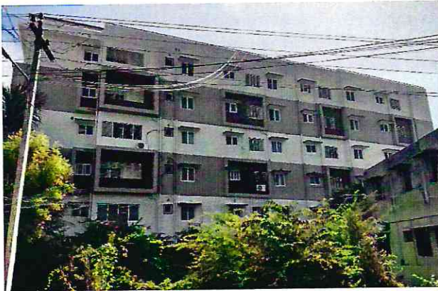
Photo taken on 15.09.2022 – East side view
