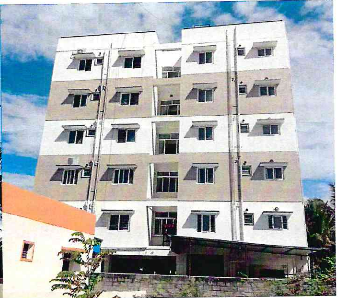
Photo taken on 15.09.2022 – North side view
