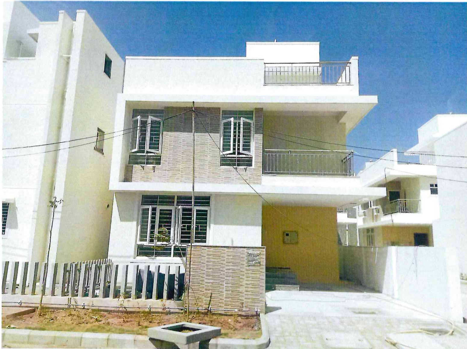
Plot No. 7A - Flooring & Painting work completed
