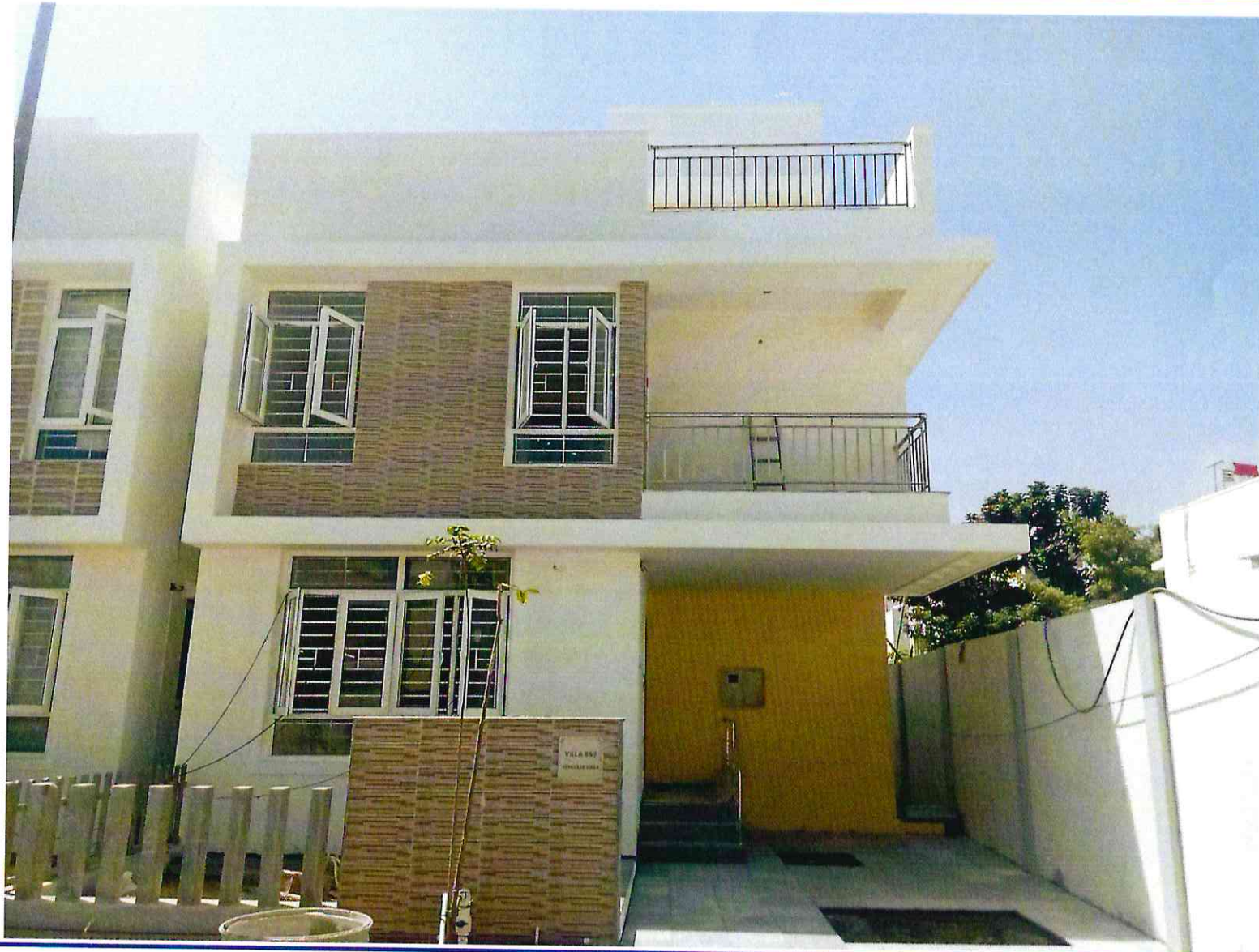
Plot No.1A - Flooring & painting work completed
