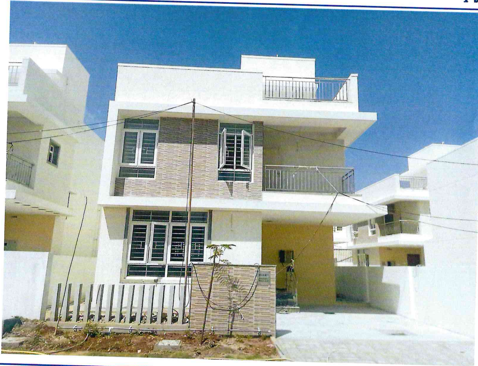
Plot No.8A – Flooring & Painting work completed
