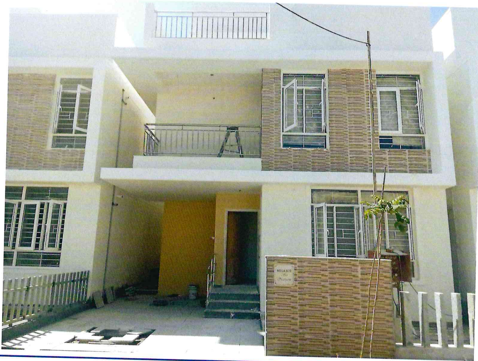
Plot No.1B - Flooring & Painting work completed
