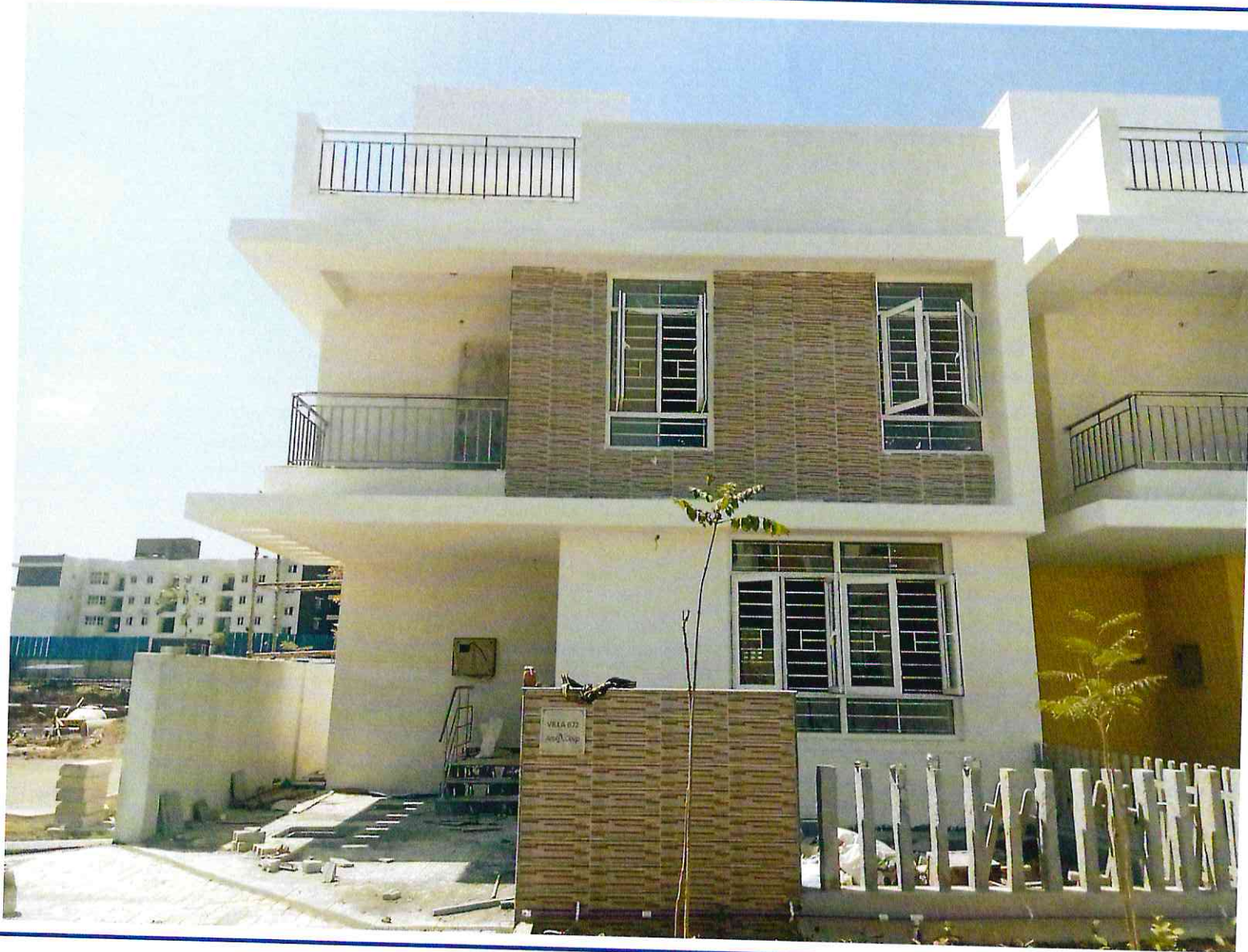
Plot No.1C - Flooring & Painting work Completed
