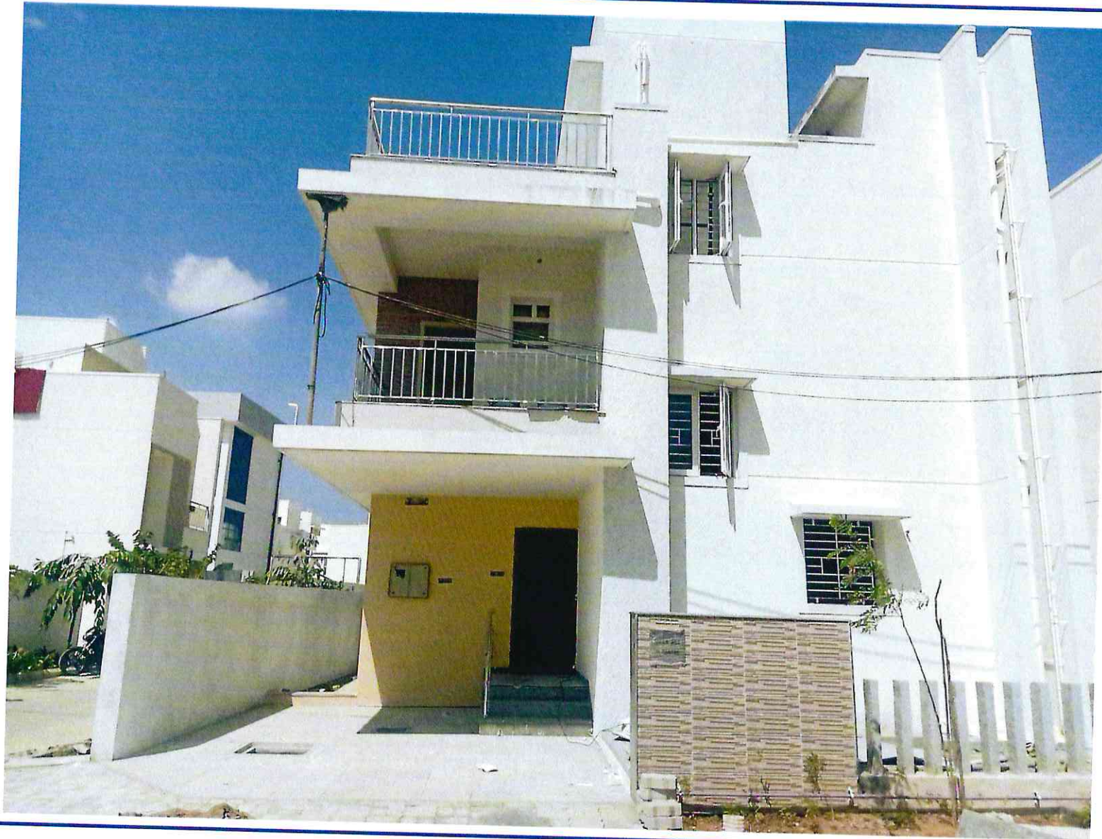
Plot No.06 – Flooring & Painting work completed
