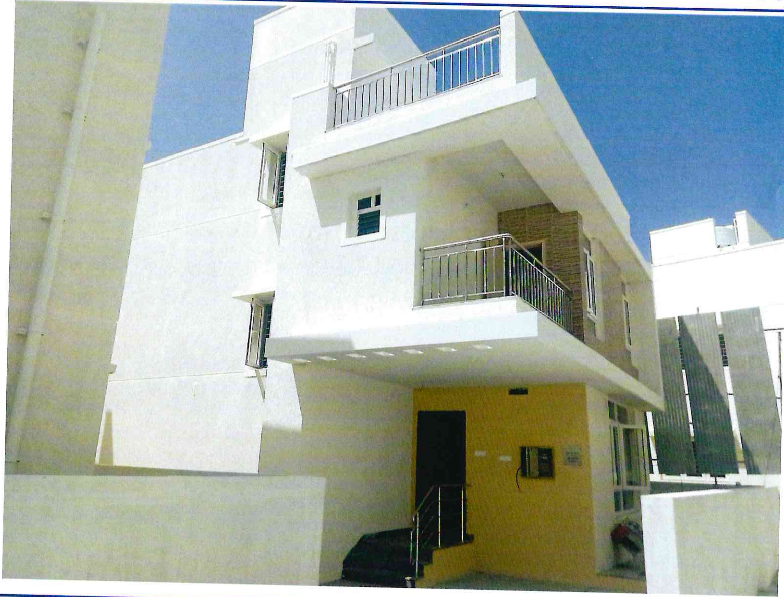
Plot No.8B – Flooring & Painting work completed
