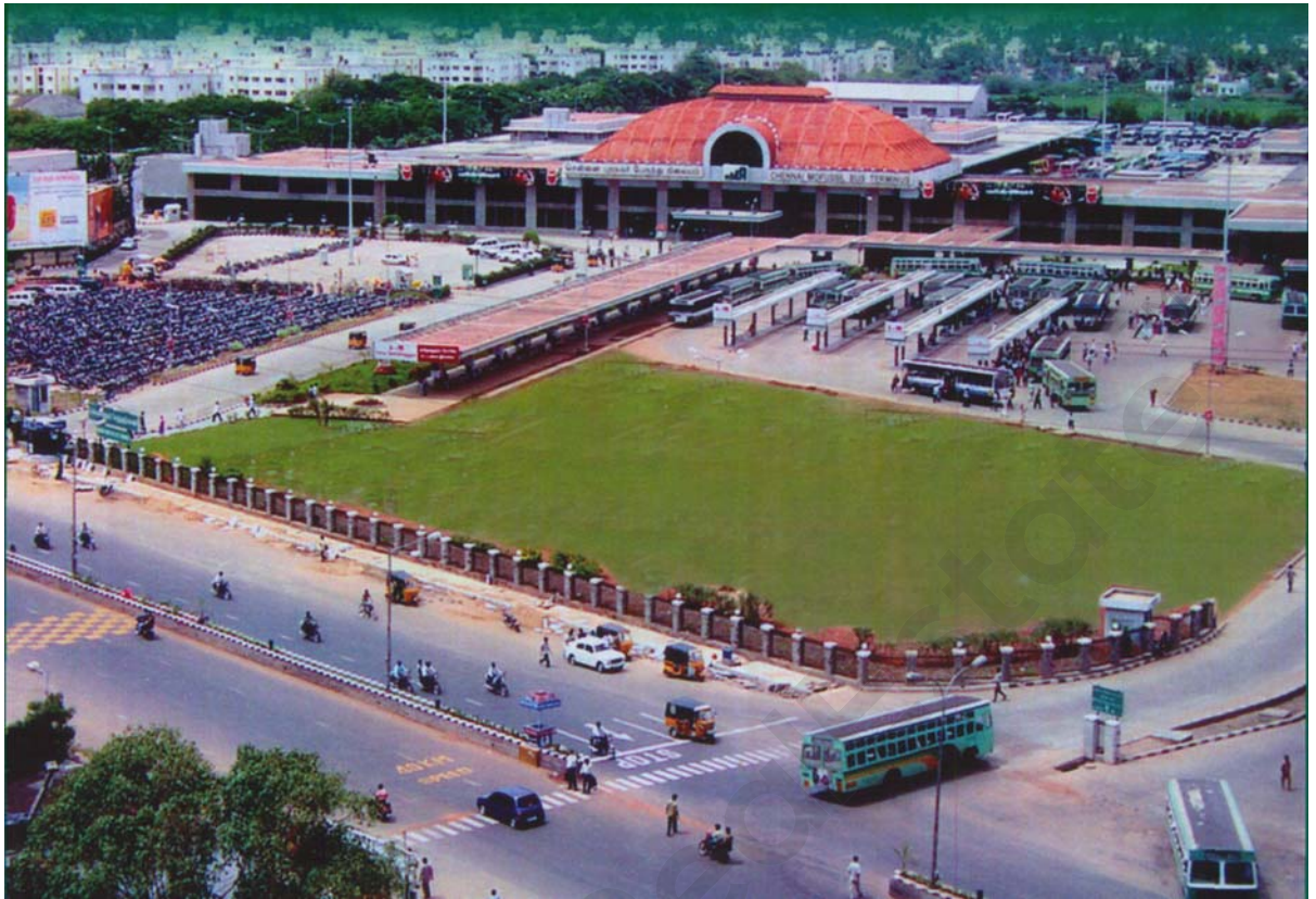
CHENNAI MOFUSSIL BUS TERMINAL AT KOYAMBEDU
