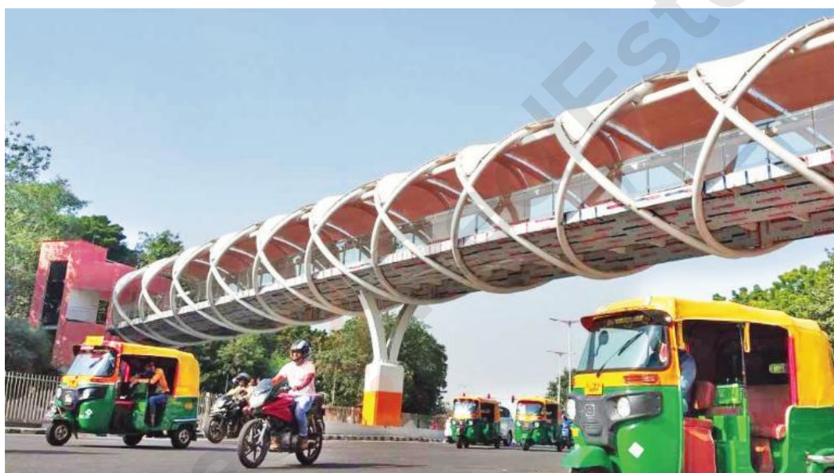
Foot Over Bridge - ITO, Delhi.
