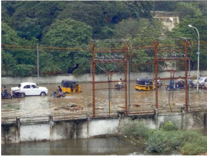
PHOTOGRAPH SHOWING THE FLOOD AND WATER LOGGING IN THARAMANI DURING DECEMBER 2005
