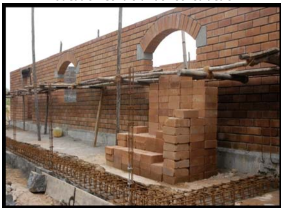
Education centre under construction
