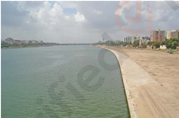
Retaining Wall and General Earth Fill
