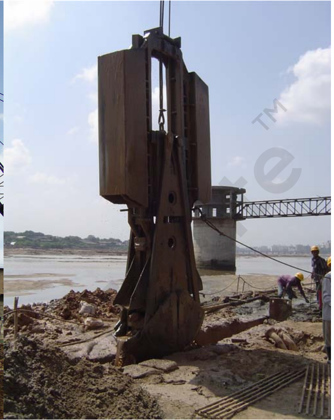
The Construction Process– Retaining Wall and Earth Fill
