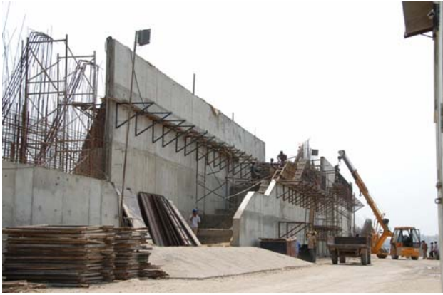
Retaining Wall and
