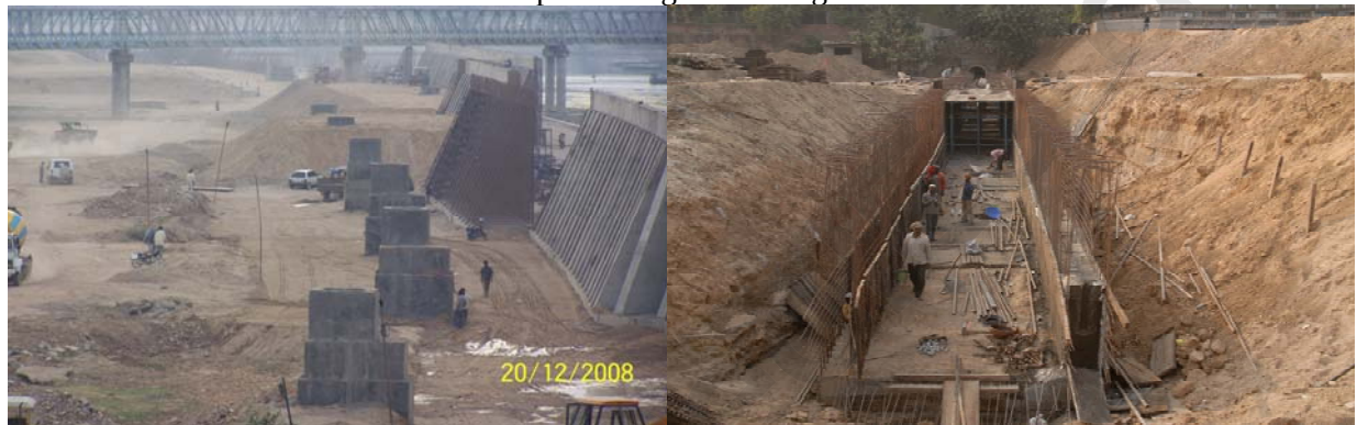
Interceptor sewage line being built
