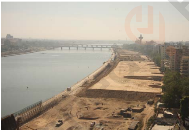
Retaining Wall and General Earth Fill
