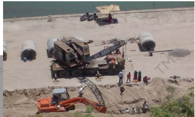
Interceptor sewage line being built
