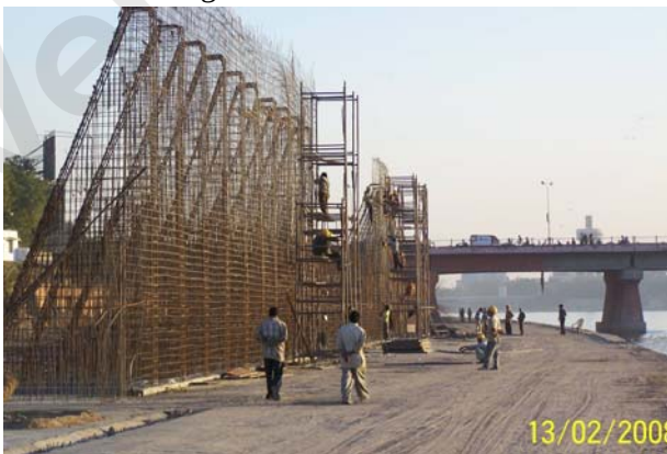
Retaining Wall and General Earth Fill
