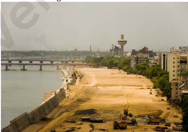
Retaining Wall and General Earth Fill
