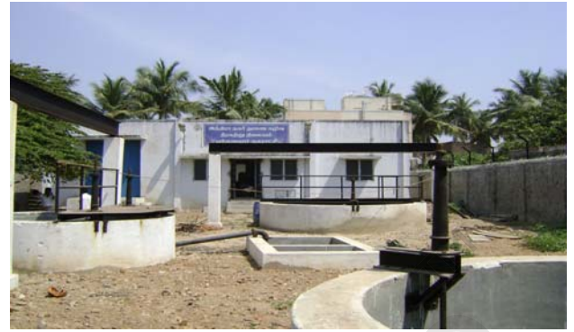
Indira Nagar Pumping Station
